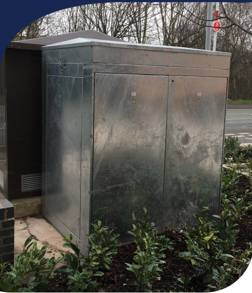
* Pillar once installed
